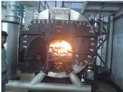
3-PASS FULLY WET BACK
